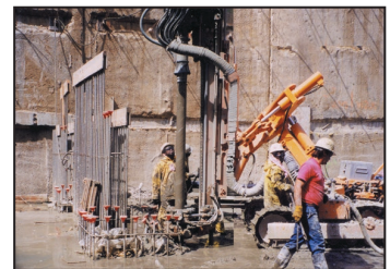
Fracturing/Regrouting
