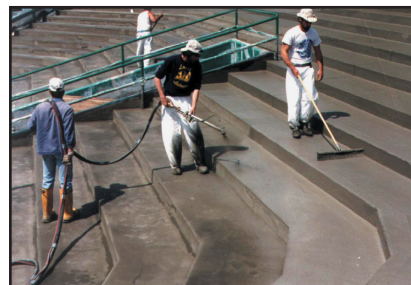
Concrete resurfacing.
