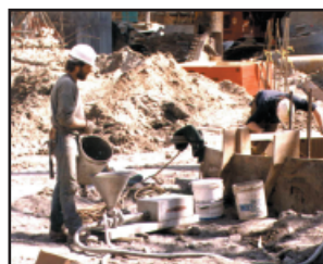
Piling Encasements
