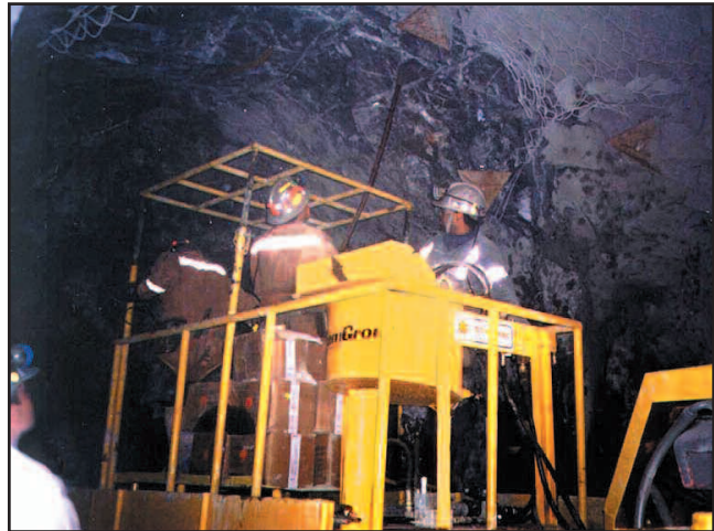
The Model 542H, shown above grouting rock bolts, is ideal for non-flowable cement grouts with water/cement ratios as low as .40 (.35 with Super "P").
