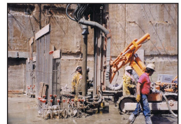
Fracturing/Regrouting
