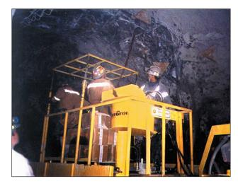
The Model 542H, shown above grouting rock bolts, is ideal for non-flowable cement grouts with water/cement ratios as low as .40 (.35 with Super "P").
