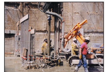
Fracturing/Regrouting
